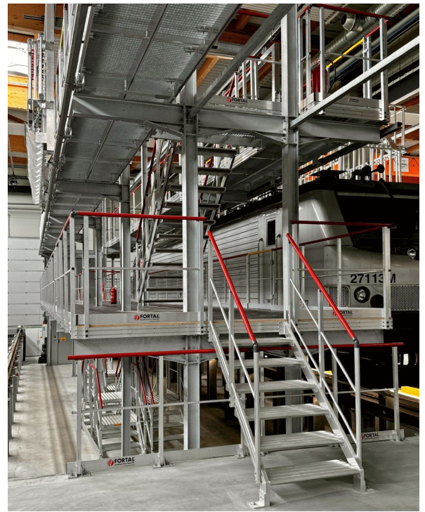
Access staircase from the train station platform
