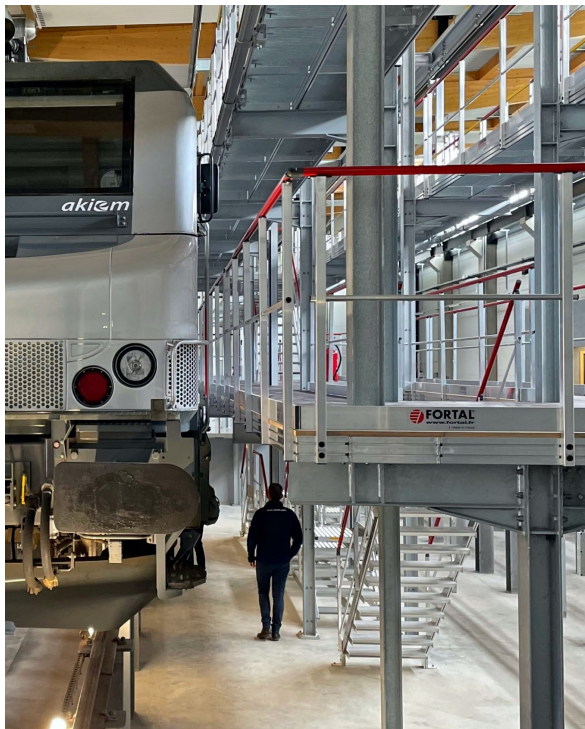
Access staircase from the bottom of the pit
